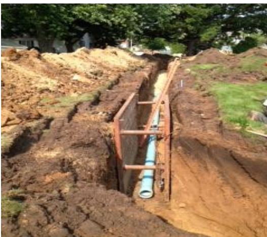
New Water Main Installation
