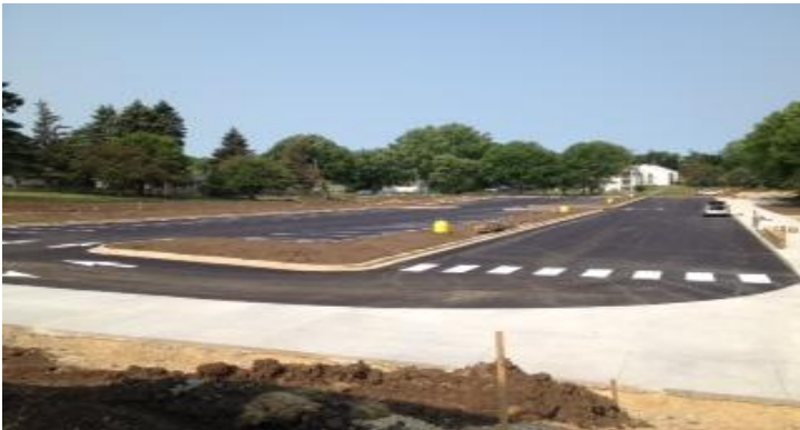
New South Parking Lot - View from East
